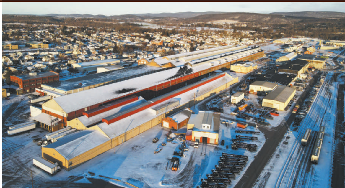
B.I.D.A. Industrial Complex today
